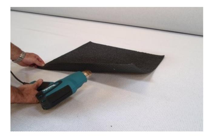
As shown on the picture you can use vinyl heat welding guns, for instance the Makita or Bosch types. This is an article which almost every carpet fitter is supposed to have, or which can be bought all over Europe.
